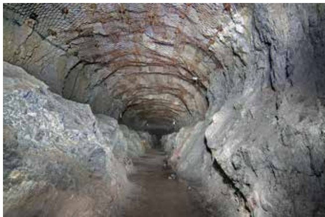
Incomplete excavations at Osowka show the crude finish to the unlined tunnels. The rock-bolted roof support is recent – installed in order to get permission for visitors to pass through. Photo Chris Wilkins
